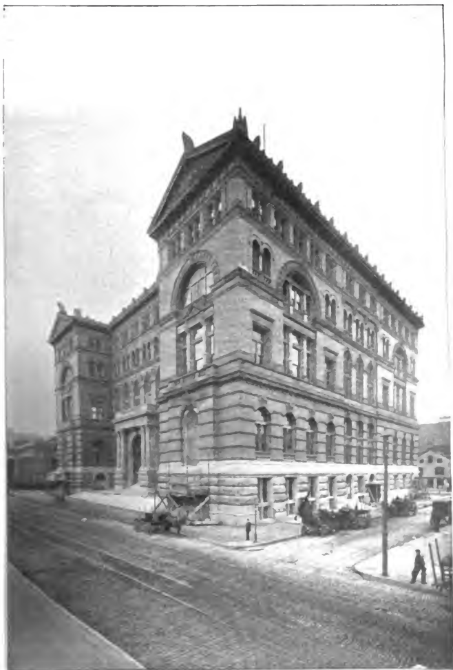
THE CRIMINAL LAW COURTS (UNFINISHED) AND THE TOMBS. CENTRE STREET, WEST SIDE, FROM FRANKLIN TO LEONARD STREETS.
